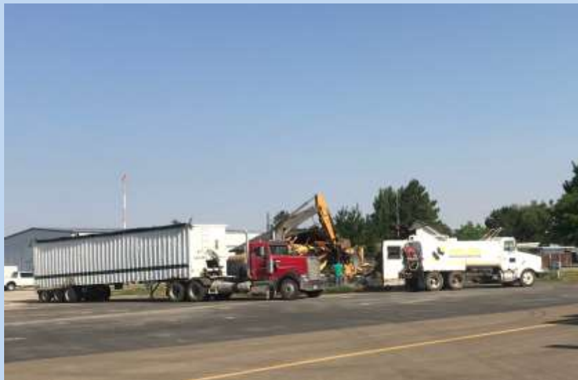
Demolition of Old FBO Demolition Video
