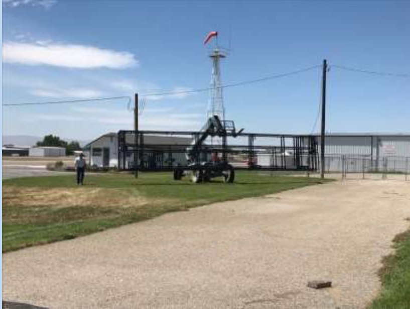
Hanger Doors being unloaded– Before Demolition
